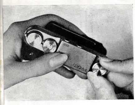
2) Set the shutter by turning the apposite knob until it stops....
